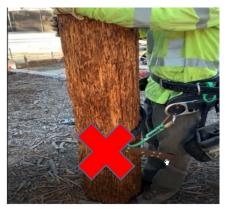
Fig. 2. Body into the pole; parallel gaffs
