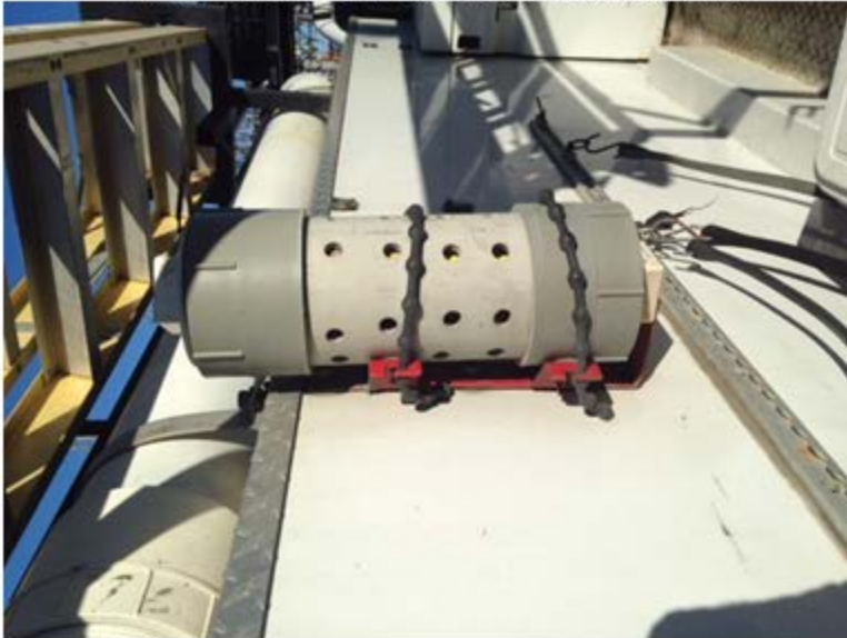
Ventilated storage of disposable propane tanks:
