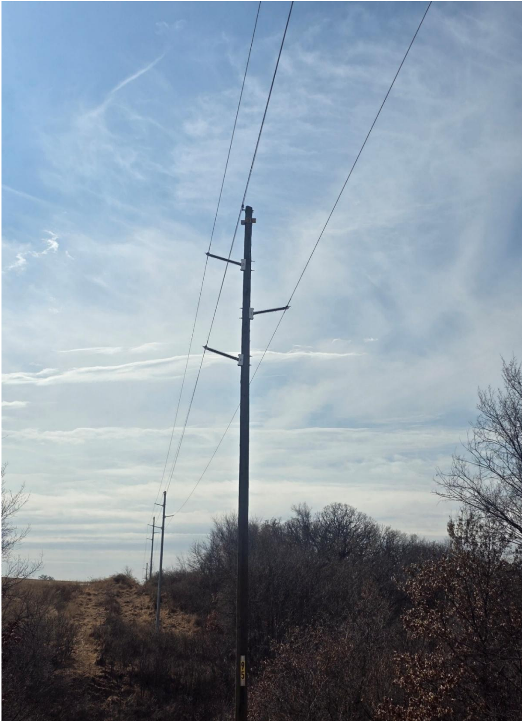
Figure 2. Vertical gain base construction
