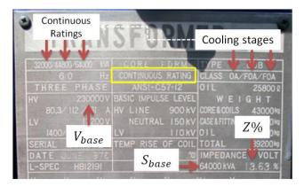
Figure 21 - Transformer nameplate
