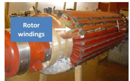
Figure 8 - Generator rotor
