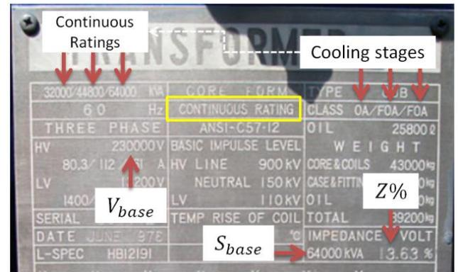
Figure 21 - Transformer nameplate
