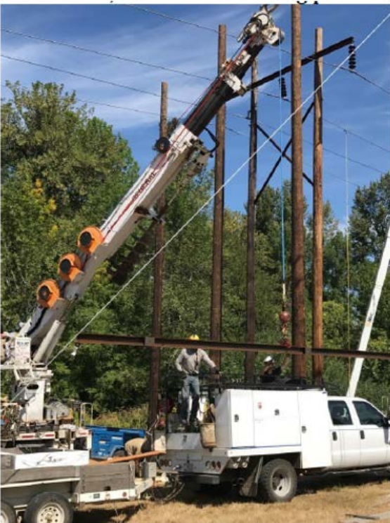
At 13:32, TLM crew 2 installing crossarm
