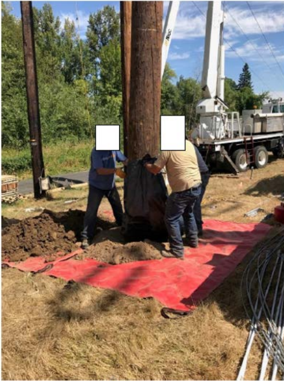
At 13:18, TLM crew 2 setting poles
