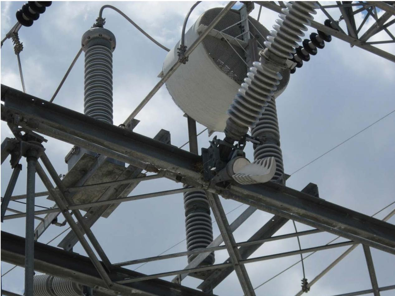
Figure 1. Remainder of Failed Vee Switch
